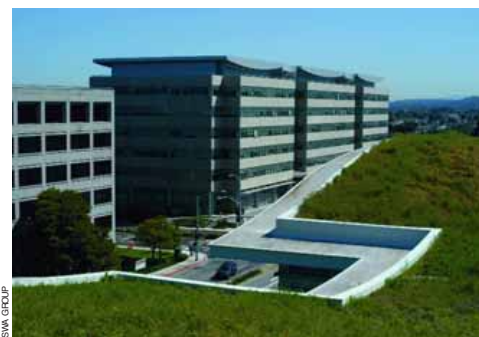
The green roof at the Gap headquarters building in San Bruno, California, conserves energy by eliminating the heat-island effect and provides a habitat for birds and insects.
