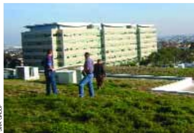
The green roof at the Gap headquarters building in San Bruno, California, conserves energy by eliminating the heat-island effect and provides a habitat for birds and insects.
