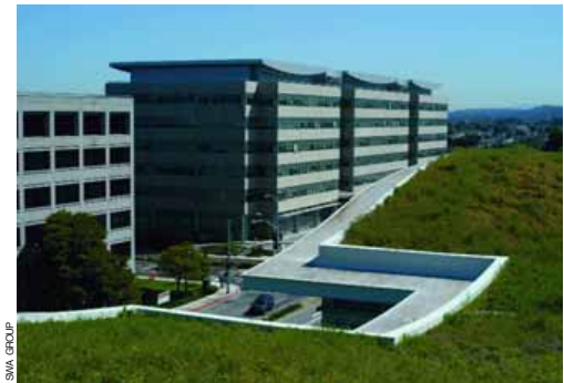
The green roof at the Gap headquarters building in San Bruno, California, conserves energy by eliminating the heat-island effect and provides a habitat for birds and insects.
